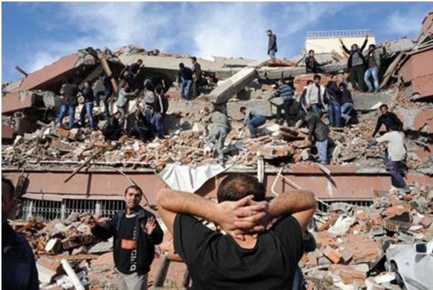
Fig. 21.1 Building collapsed during the 2011 Van Earthquake in Turkey (Courtesy of National Turk)
