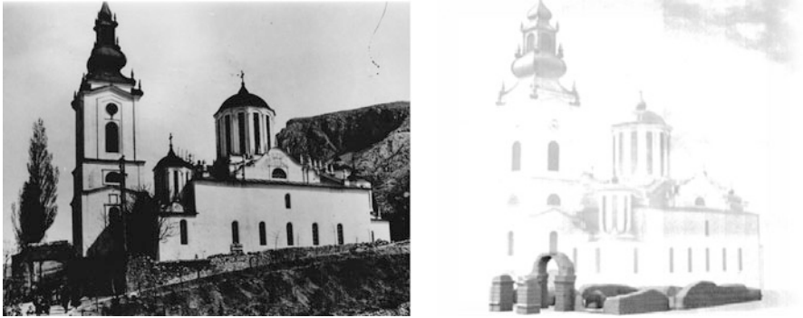
Fig. 8.19 The original Holy Trinity church in Mostar and view of the torn down church
