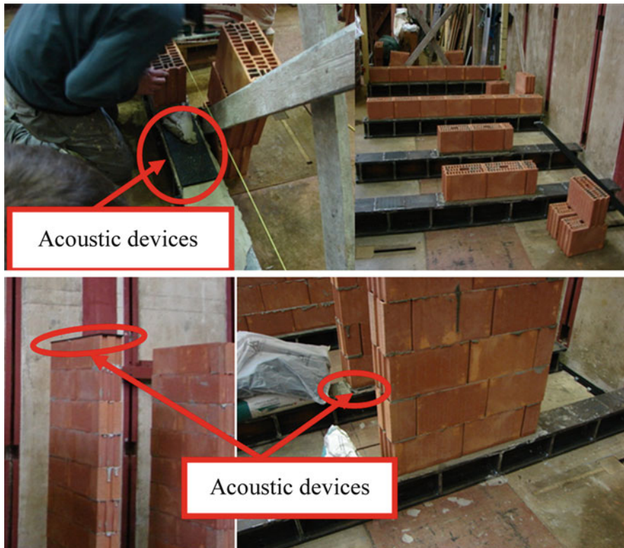
Fig. 6.1 Wall specimens with soundproofing devices at top and bottom
