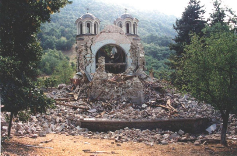
Fig. 8.13 The church after detonation
